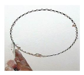
3-Fish the speaker cable from the amplifier and out through the recently cut speaker cavity. Allow yourself roughly 1' (30cm) of slack to protrude to facilitate the installation. Strip about 3/8" (1cm) off the ends of the speaker wires and connect to the speaker terminals.
